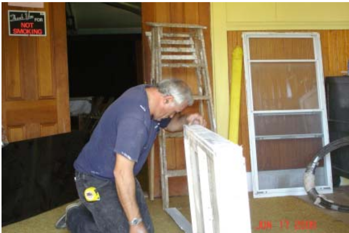
Norman Vashon preparing a replacement window
