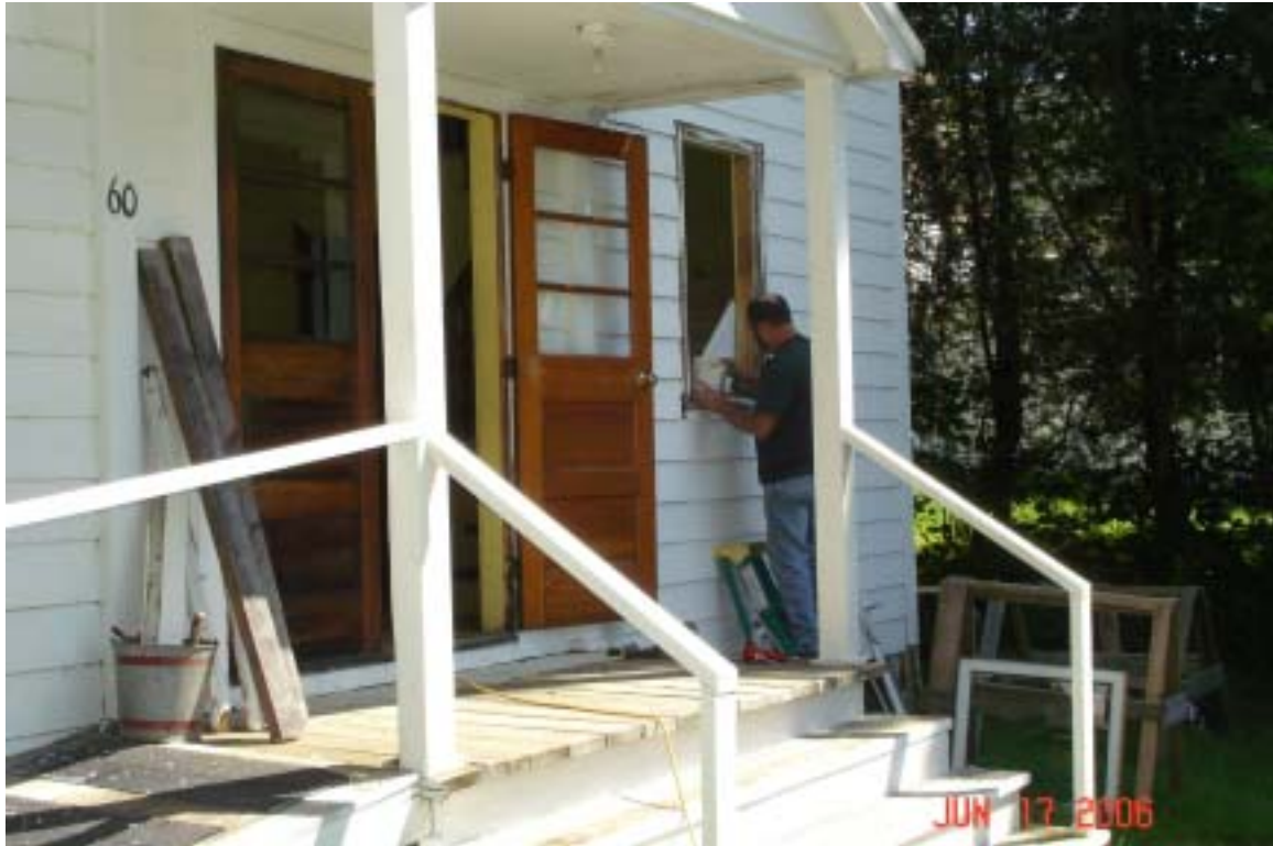
Clyde Rolerson working on a window
